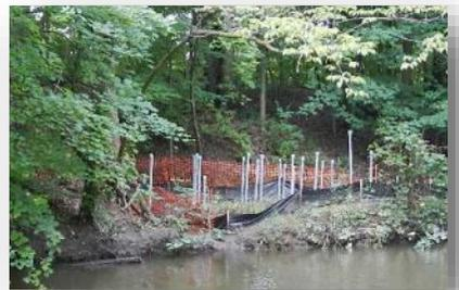
In early July, the contractor started work on Ellsworth Boardwalk. Up went the orange fence and the black silt fence. Plenty of stakes and paint marked the site. The pathway was cleared and materials stacked.
